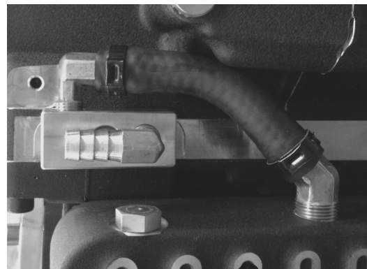
STRAIGHT LINE INSTALLED, FIGURE 7
